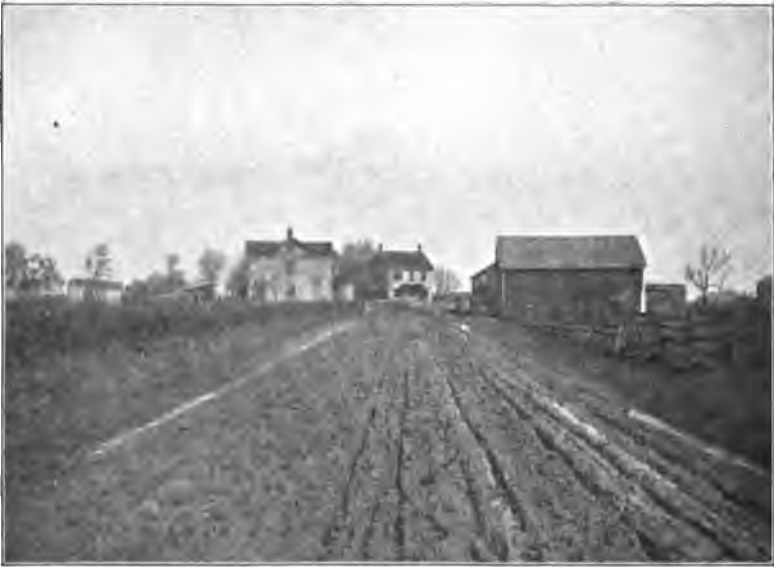
Neshanic road, Somerset Co., before improvement.
